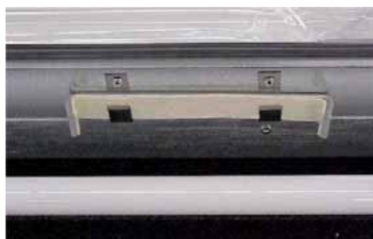
Illustr. 5-5 Suspension of the base pane
