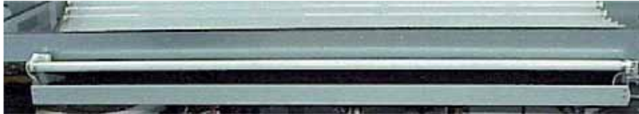
Illustr. 5-17 Filter mat in the base section
